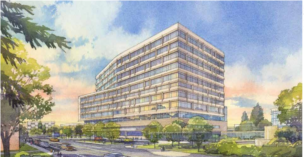
Top 150 Distributors are working on some very large hospital projects. One of the largest is the Pavilion at University of Michigan Health. The 12-story hospital will house 264 private rooms capable of converting to intensive care; a state-of-the-art neurosciences center; and advanced imaging facilities.
